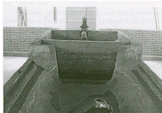
Fig. 3. The inlet part of the flume and the basin.
